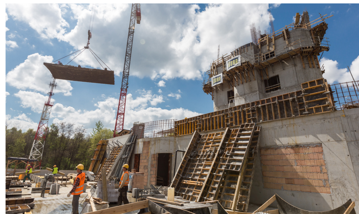
Construction works of TWR in Cracow
