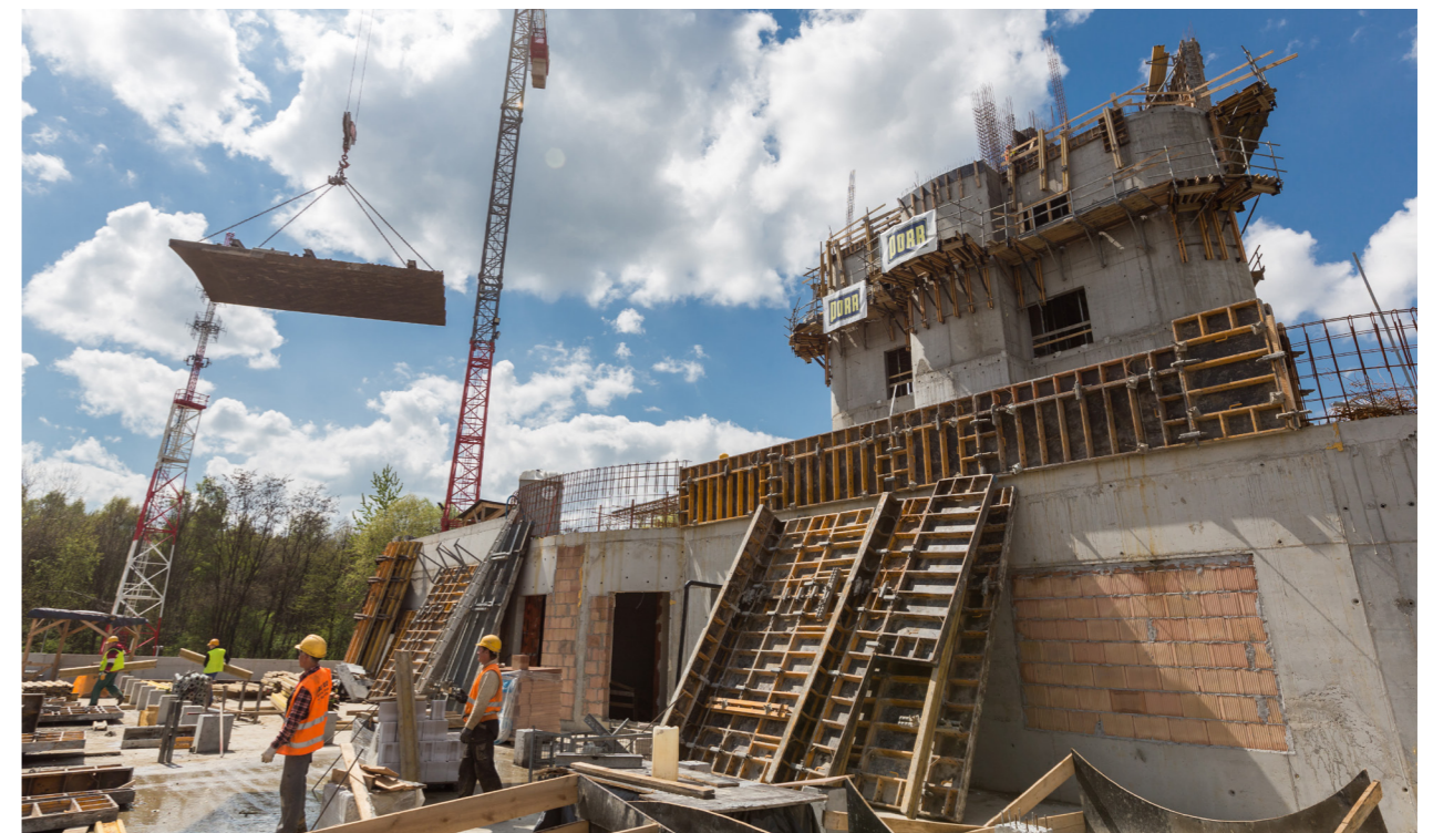
Construction works of TWR in Cracow
